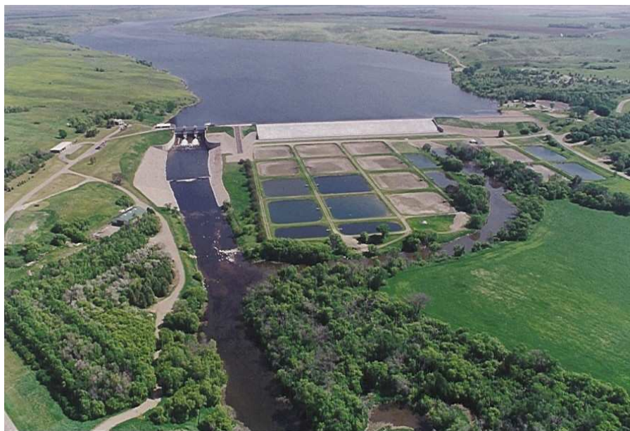
1944: Baldhill Dam, Sheyenne River
