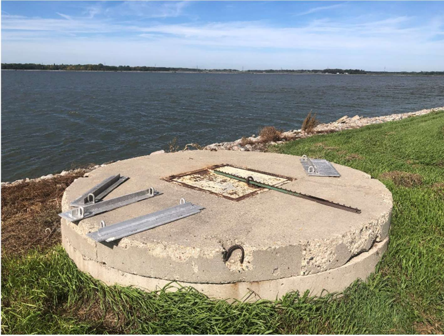
Figure 4. Cell # 2 of the Thief River Falls Wastewater System.
