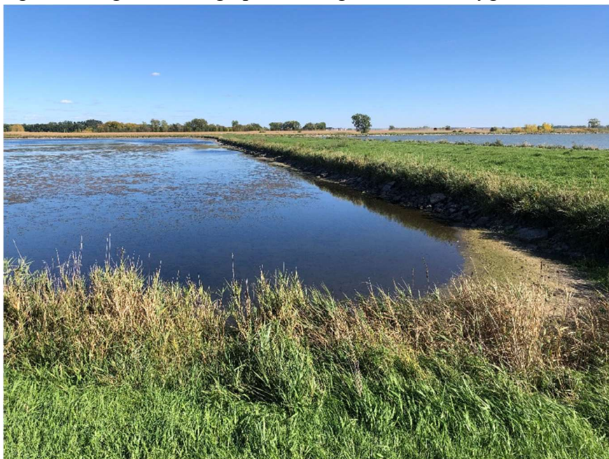
Figure 3. Cell # 2 of the Mahnomen Wastewater Lagoon System
