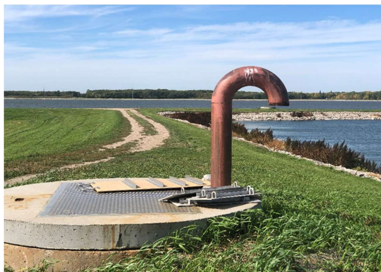
Figure 2. Cells 1 & 2 of the Thief River Falls Wastewater Lagoon System
