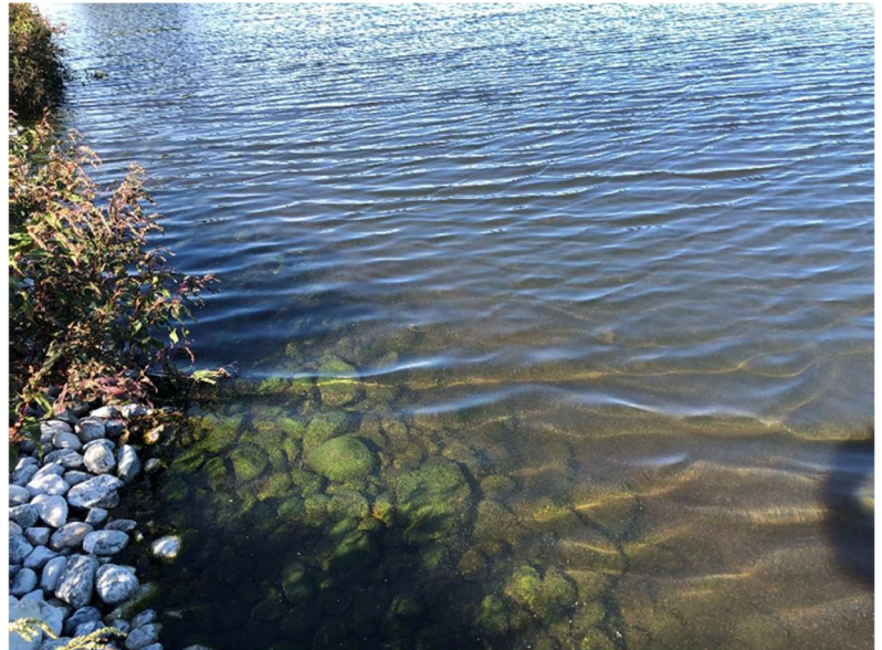
Figure 5. Cell 4 of The Mahnomen Wastewater Lagoon System
