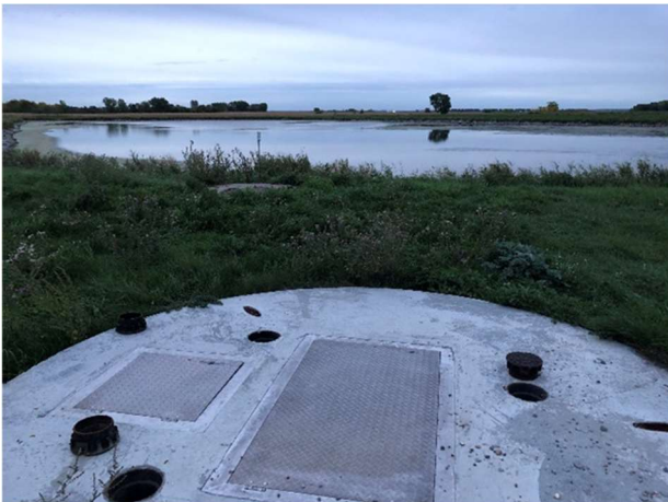
Figure 2. Cell # 4 of the Mahnomen Wastewater Lagoon System.
