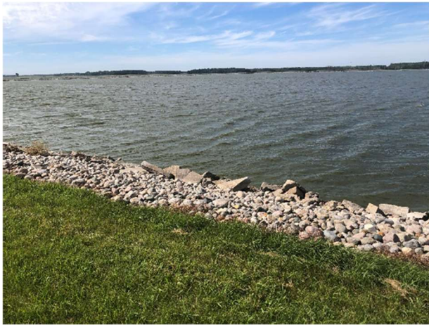
Figure 3. Cell # 3 of the Thief River Falls Wastewater Lagoon System.
