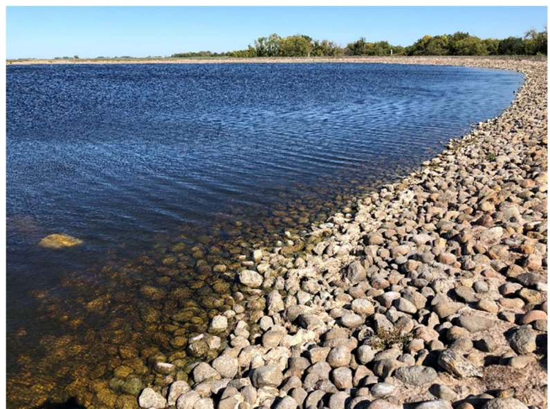
Figure 5. Cell # 3 of The Hillsboro Wastewater Lagoon System. Water in this cell is exceptionally clear.
