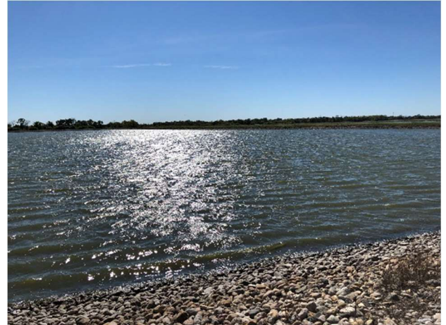
Figure 3. Cell # 1 of the Hillsboro Wastewater Lagoon System.
