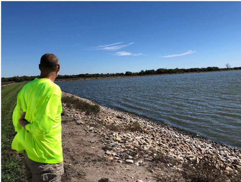
Figure 4. Operator Mike Hovet Looking at Cell # 2 of the Hillsboro Wastewater System.
