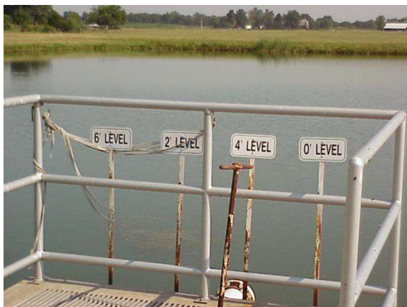
Figure 5. Pulling the Water Below Three (3) Feet Will Generally Result in Fewer Algae Cells Being Discharged
