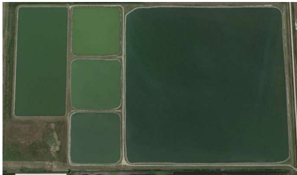
Figure 1. The Five Cell Breckenridge Minnesota, Facultative Wastewater Lagoon System
