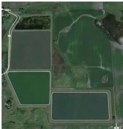
Figure 1. The Mahnomen Minnesota, 4-Cell Facultative Wastewater Lagoon System
