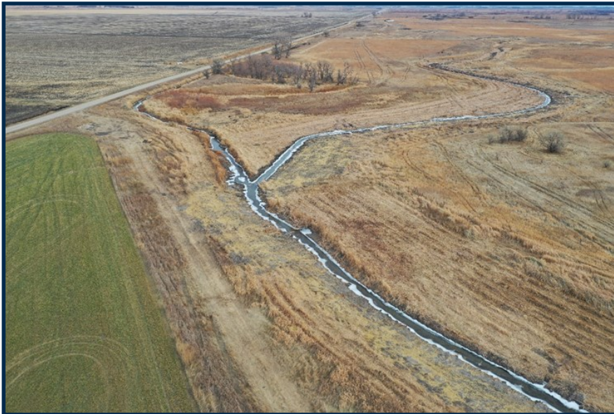
Aerial view of the project site during construction in 2022.
